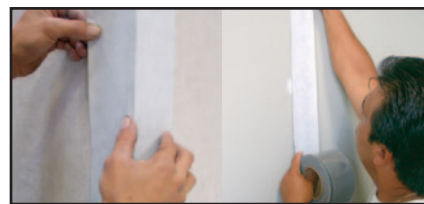
APPLY MULTICOAT ELASTOMERIC JOINT TAPE TO CORNERS AND JOINTS
